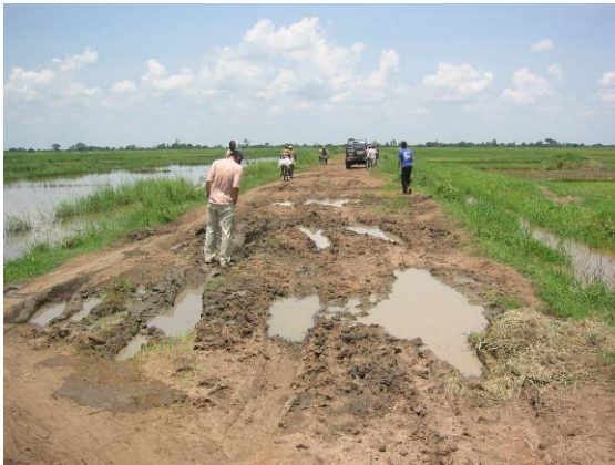
Figure 1. A rural road in the rainy season, via which rice is transported (Uganda)
