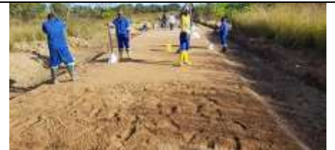
Picture6: Covering and final compaction
