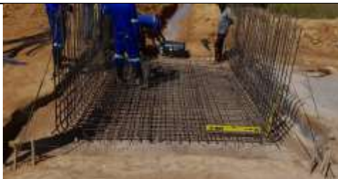
Picture10: Fixing The confirmed Iron bars bottom slab of bridge
