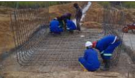
Picture11: Tying the iron bars
