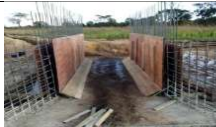
Picture 14: Shuttering process with plywood
