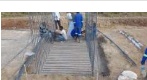
Picture13: Distribution bars fixing on the wall of box culvert
