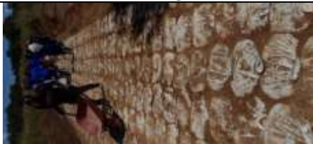
Picture 4: Filling the gaps between each four compacted Do-nou bags
