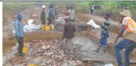
Picture8: Base foundation for box culverts
