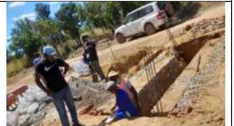
Picture 15: Wall bridge masonry constructed at kamiba
