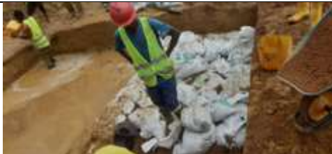
Picture7: Soft soil foundation stabilization with Do-nou bags
