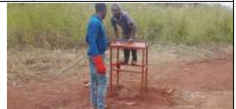
Picture 9: Iron bars bending to the fixed measurements
