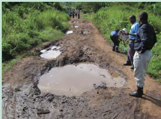
Before (道直し作業前)
